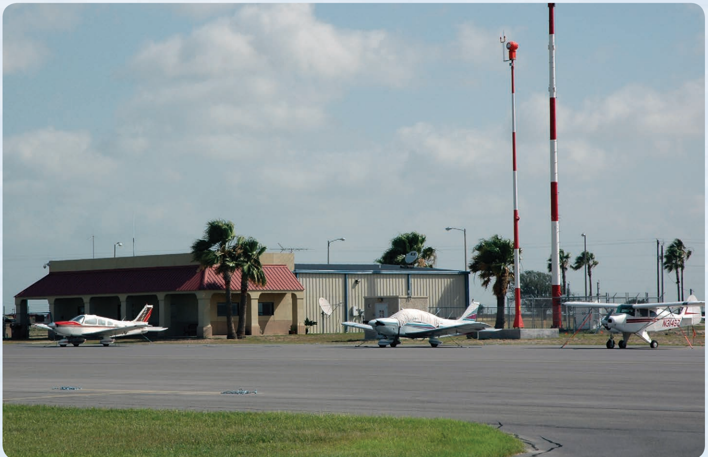
The terminal building at South Texas International Airport at Edinburg.
