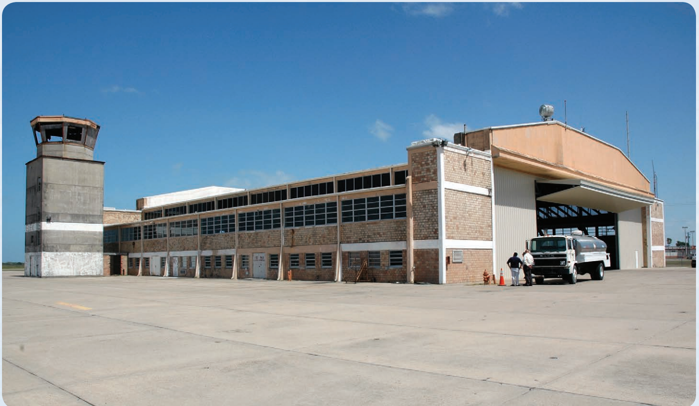
The historic hangar at Port Isabel-Cameron County airport with its new door retracted. Future plans include refurbishing the adjacent control tower.
