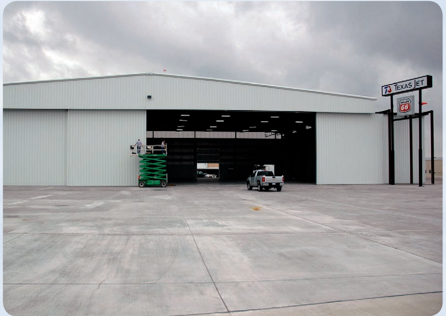
The rebuilt Texas Jet hangar at Fort Worth Meacham Airport. The original hangar was destroyed in a storm in 2012.
