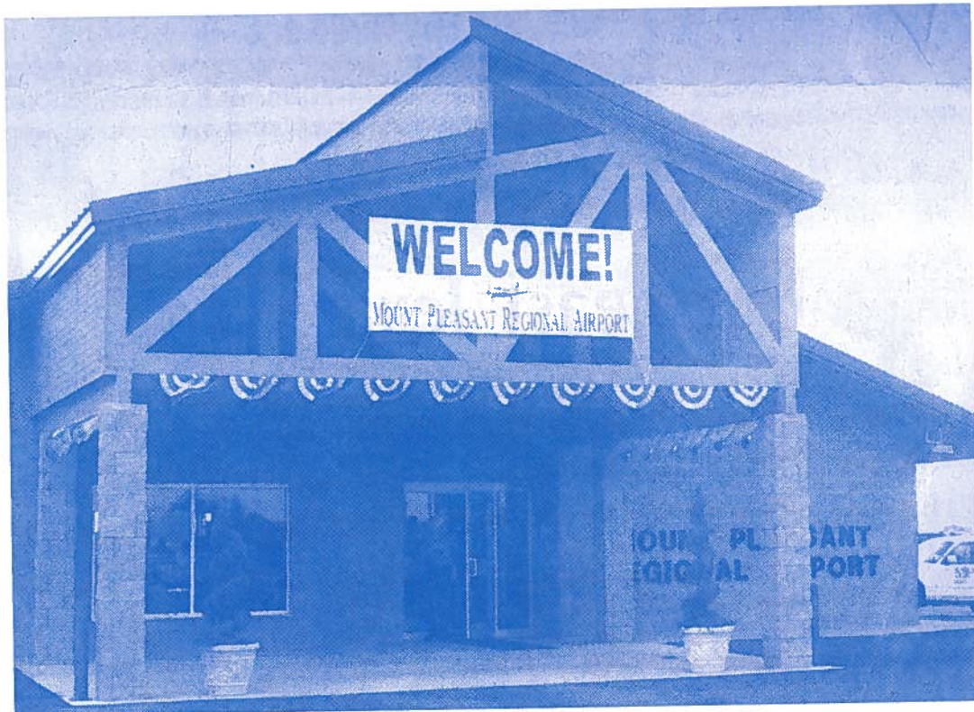
MOUNT PLEASANT REGIONAL AIRPORT - New terminal building dedicated last fall.
