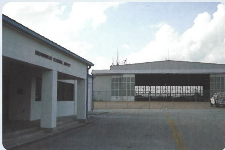
Terminal and large hangar facility at Brownwood Regional Airport.
