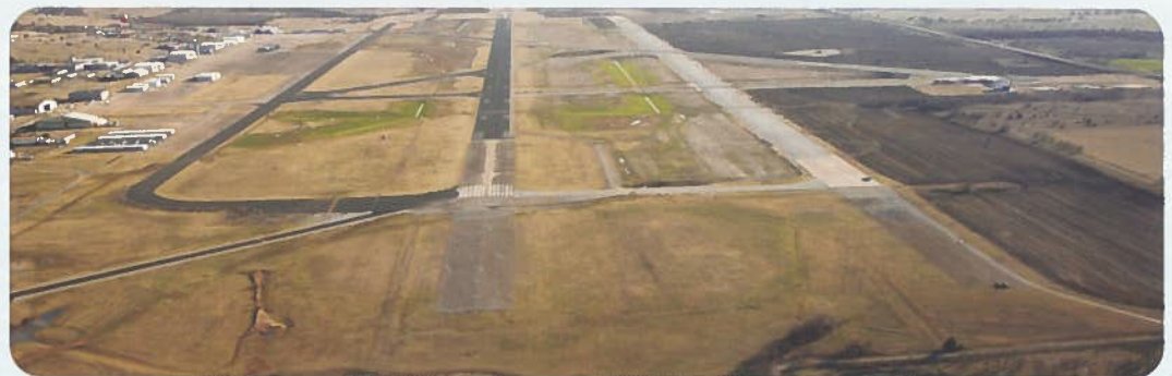
Room to grow: The expanse of the North Texas Regional Airport is evident in this aerial photo. The construction of State Highway 289 can be seen on the far right.
