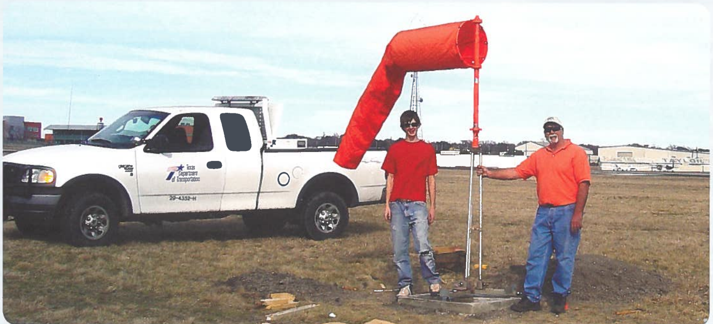
Tommy Waldo and Alton Young stand beside the newly constructed windsock for the Taylor Municipal Airport. Alton, an Eagle Scout, helped Tommy earn his Eagle Scout with this project.
