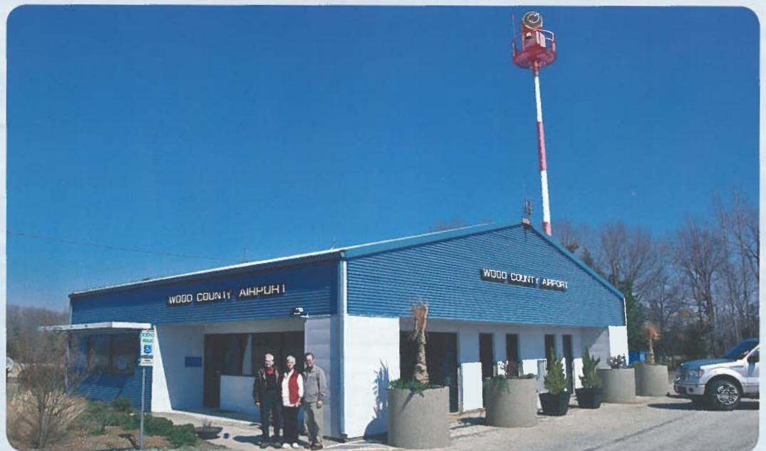
Wayne Collins, Sandra Braden of TxDOT Aviation and Dr. John Wisdom in front of the Wood County Airport terminal building.
